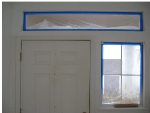
FIG. 2: OPENINGS PREPARED FOR PAINTING, WITH PLASTIC SHEETING.
