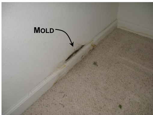
FIG. 3: APPARENT BLACK MOLD AT WATER SPOT
