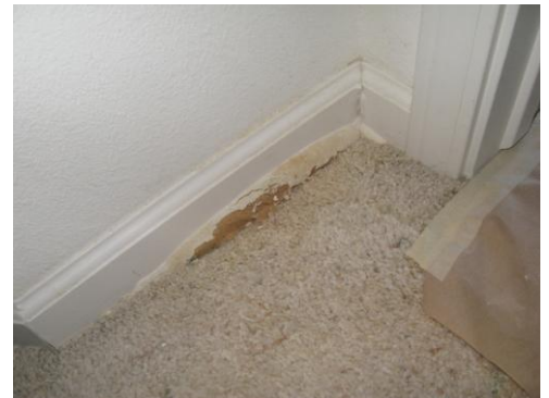
FIG. 8: WATER DAMAGE AT BASEBOARD.
