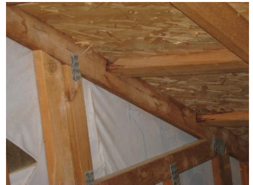
FIG. 7: WATER DAMAGE AT OUTLOOKERS.
