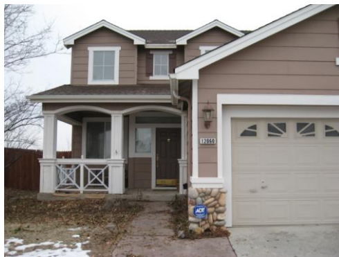
FIG. 1: EXTERIOR OF RESIDENCE
