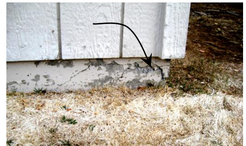
FIG. 5: CONCRETE DEGRADATION.
