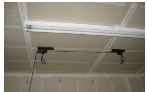
FIG. 6: CEILING MOUNTED LIFT HOOKS
